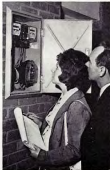
Right: Norma with Mr. Ron Williams (District Commercial Engineer) doing a check reading on the meters installed in a box unit outside the entrance to each flat.
